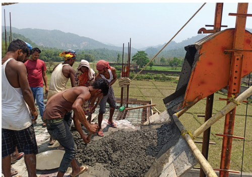
9. SLAB CASTING
